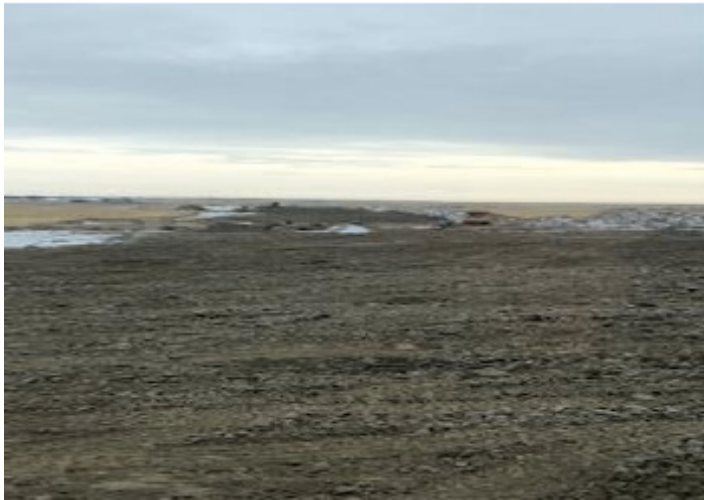
Reclaiming natural grade - km 169+455 – Nov 9, 2018
