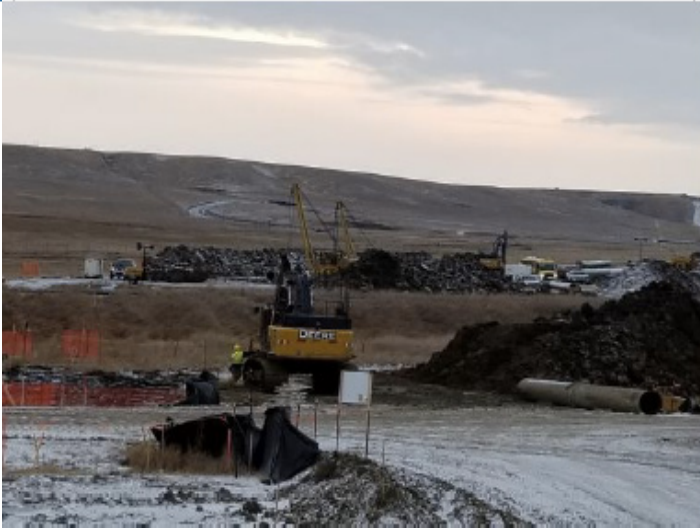
Bore crew- km 221+150 – Nov 10, 2018
