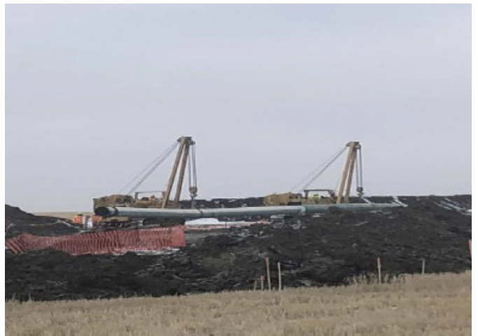
Tandem lift for tie-in – km 197+500 – Nov 6, 2018
