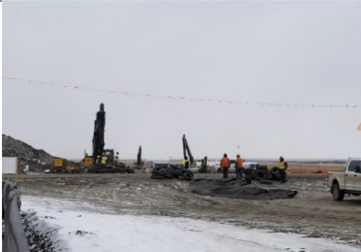
Getting ready to cross equipment – km 259+200 – Nov 7, 2018
