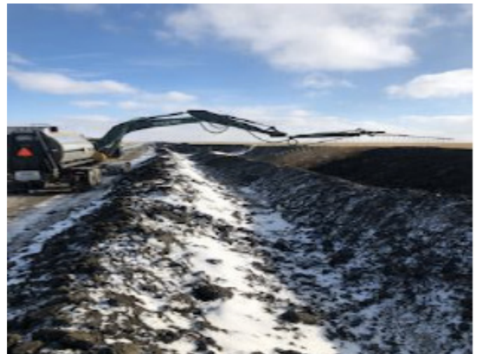
Excavator spraying piles– km 246+375 – Nov 6, 2018
