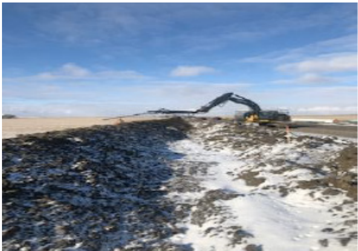
SITE crew spraying tackifier– km 259+800– Nov 8, 2018
