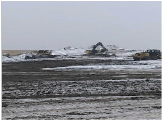
Excavator loading rocks – SF 101 – Nov 8, 2018
