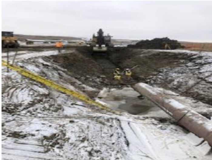
Digging tie-in ditch – SF 140 – Nov 10, 2018
