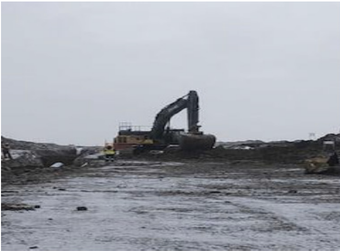
Excavator shading pipe for final tie-in – SF 112 – Nov 8, 2018
