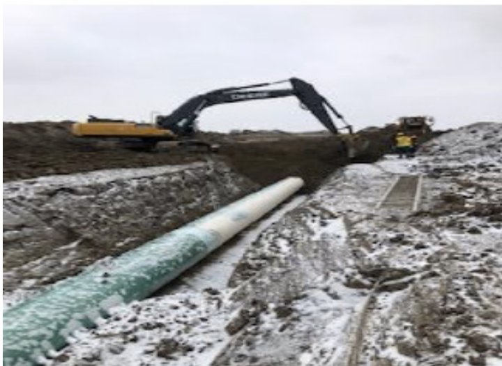
Tie-in backfill – km 175+170 – Nov 7, 2018
