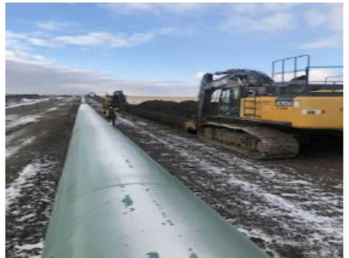
Digging mainline ditch – km 238+750 – Nov 8, 2018
