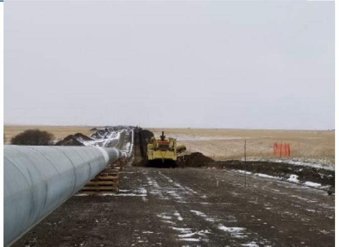
Digging the ditch – 236+070 – Nov 7, 2018
