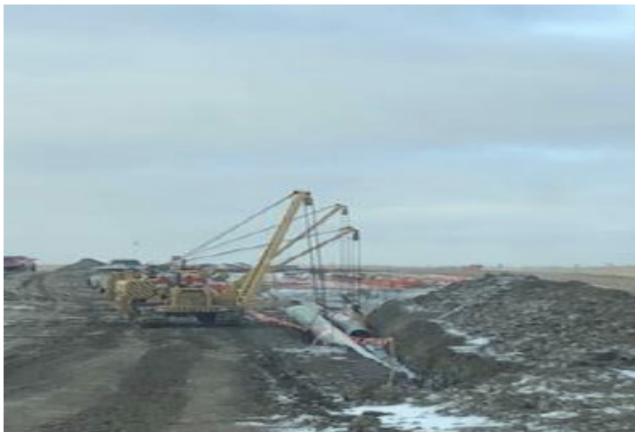
Welding crew and final tie-in – Km204+800 – Nov 6, 2018
