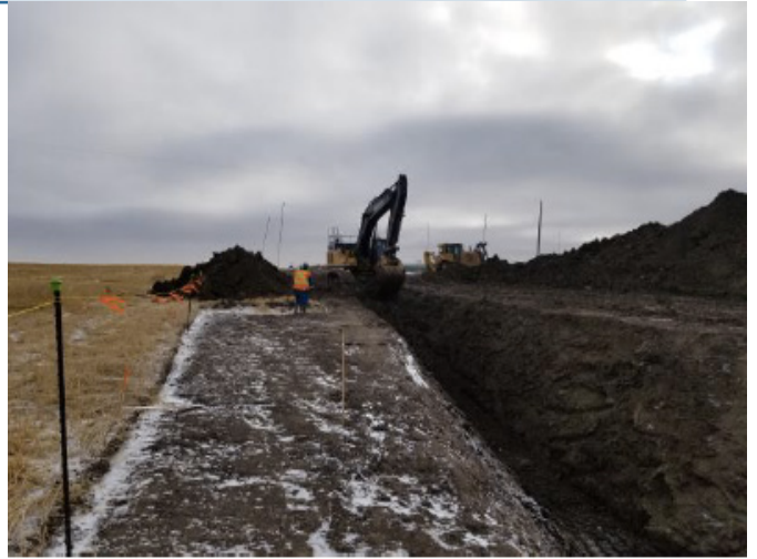
Digging tie-in section – km 197+500 – Nov 6, 2018
