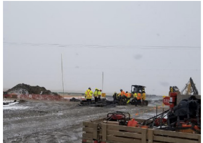
Crossing equipment– km 224+743 – Nov 5, 2018
