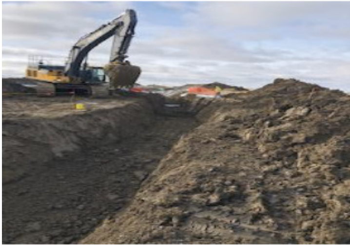
Backfill crew pulling soil - km 222+370 – Nov 5, 2018
