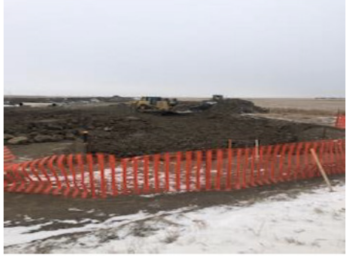
Tie-in backfill crew – SF 113 – Nov 9, 2018
