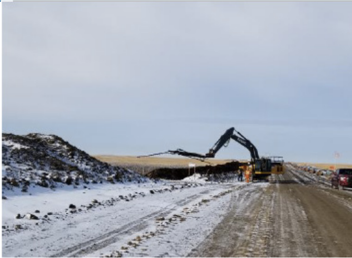
Tackifying soil – km 263+500 – Nov 9, 2018
