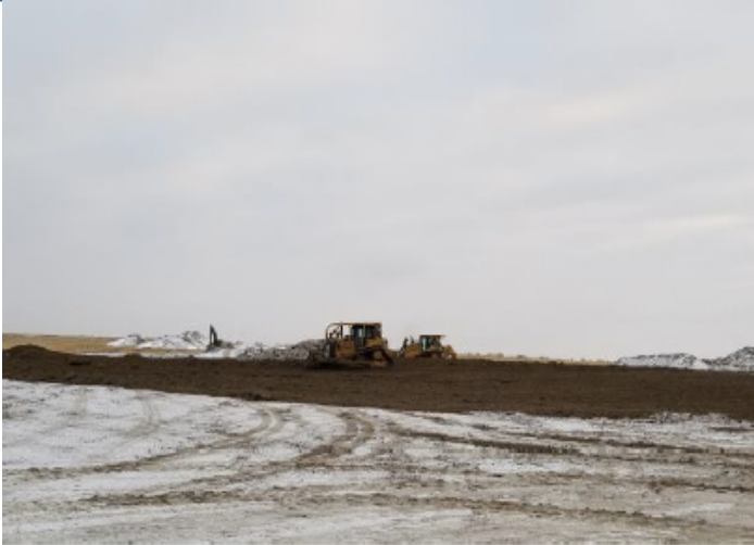
Grading ROW – km 170+940 – Nov 8, 2018
