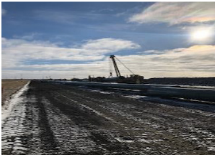
Bending crew pulling bends – km 211 – Nov 6, 2018
