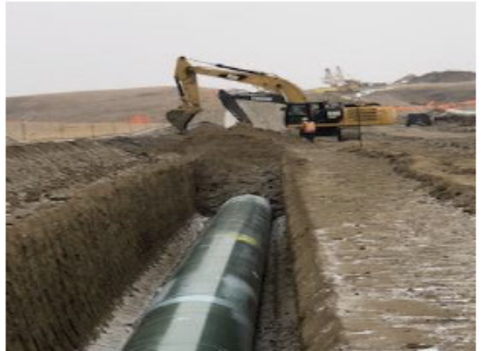
Tie-in excavator - km 197+360 – Nov 5, 2018
