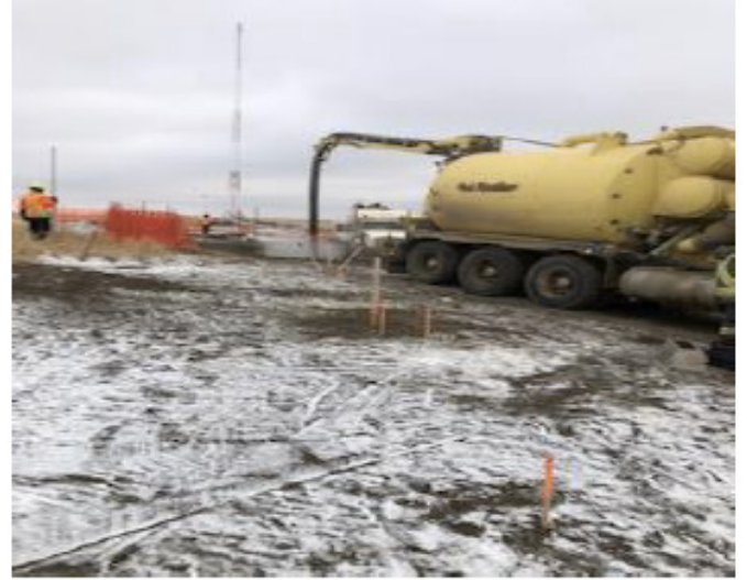
Hydrovac slot digging – km 209+703 – Nov 10, 2018
