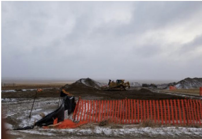
Moving dirt – km 172+100 – Nov 5, 2018
