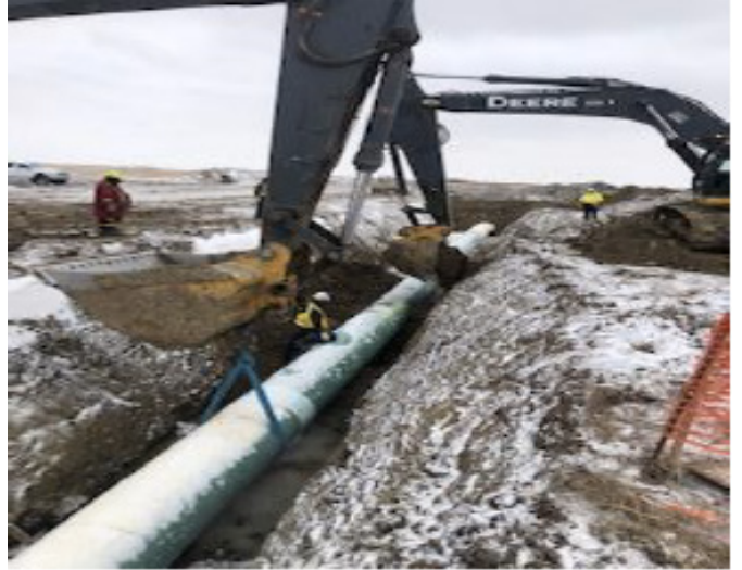
Excavator shading pipe at Plains mainline crossing – Nov 7, 2018
