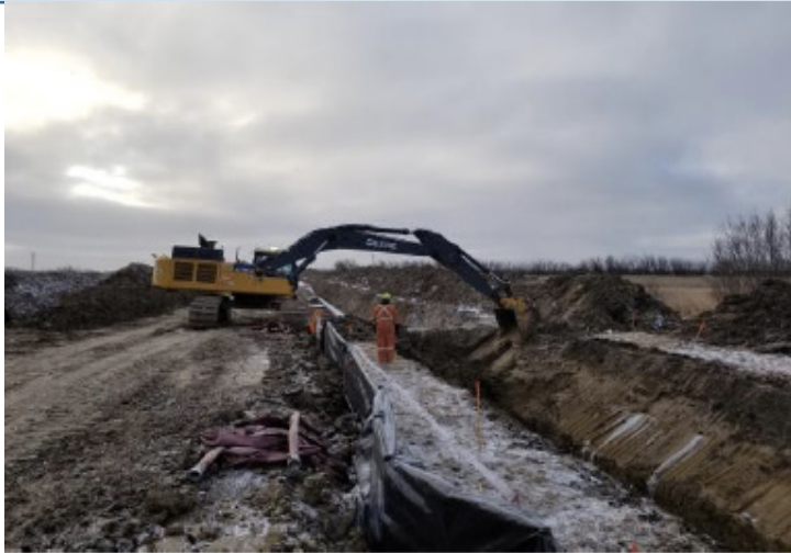
Digging ditch for tie-in – km 180+100 – Nov 6, 2018
