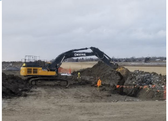
Shading tie-in section – km 197+400 – Nov 8, 2018
